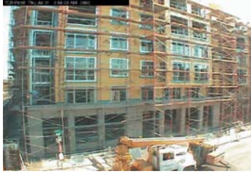
10th@Hoyt Development Pearl District of Portland, Or.
